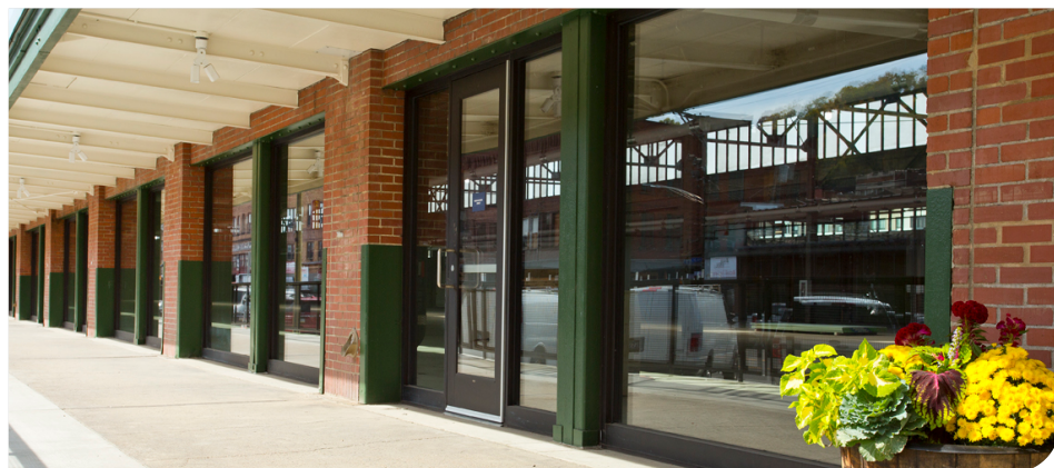
Solarban® 72 and Acuity™ glasses deliver transparency, color-neutrality, solar control and visible light transmittance for the revamped Pittsburgh Produce Terminal.
